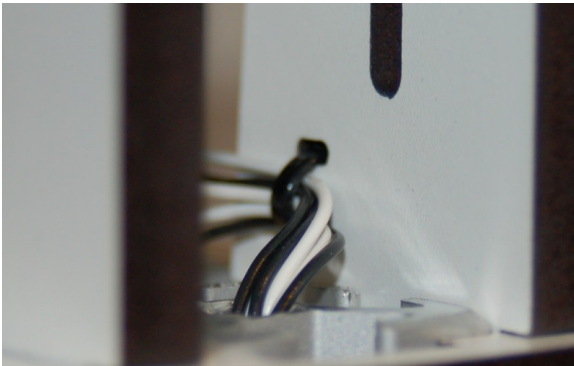
Fig. 7-40: End stop wires pulled tight.
