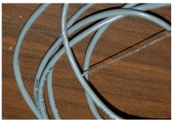
When you're done, you can discard the outer jacket and the thin aluminum wrap. However, don't discard the bare wire that was woven around the four conductors. You're going to use that shortly as a pull line to get the thinner wires down the towers.
